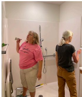
Centenary UMC volunteers painting a bathroom inside the Lynchburg home
